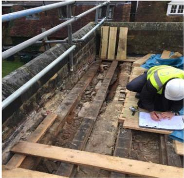
A tin roof is now sitting on the south roof of St Dunstan's in Mayfield. It was not planned to be there but work expected to finish by Christmas, revealed serious structural problems with the old beams, caused by death watch beetle. Structural engineers have drawn up a remedial plan, and the tin roof has arrived to allow the skilled workmen to do their job in
